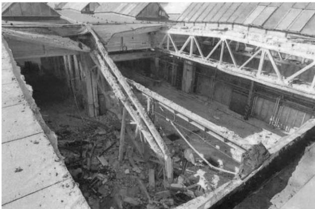
Figure 2 – Failure of roof trusses in industrial hall
