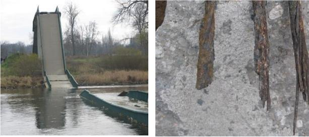
Figure 1 – Collapse of Prague footbridge and total damage of its prestressing reinforcement
